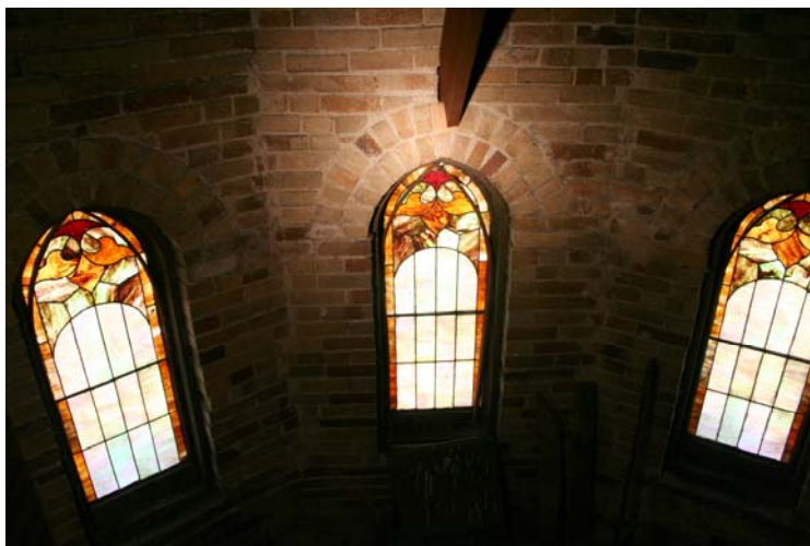
Windows above entrance. Each one is 17"x by 50".
